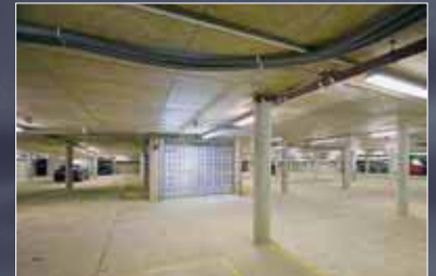
Typical underground car park
